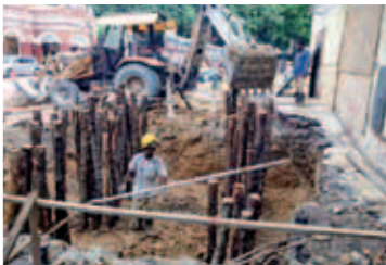
Bakau Pile in progress at link bridge
