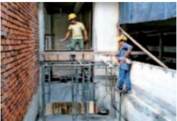
Staircase 4 fwk installation at mezz 1 st floor in progress
