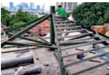
Welding work Asuka Tower roof truss in progress
