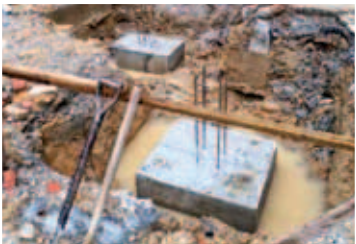
Footing completed nos at link bridge
