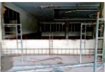
Lintel beam & stiffener in progress at Mezz Floor
