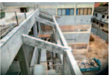
Lower Roof Beam completed pending for roof truss
